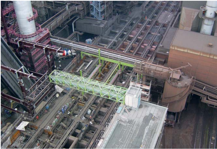
Figure 1. Elevated railway bunker unit (without dust capturing unit)
